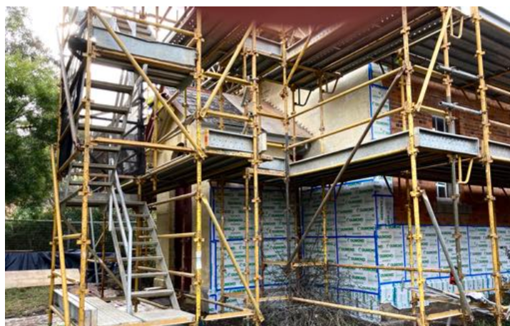
Eltham Courthouse under restoration Photograph - Jim Connor - July 2021
